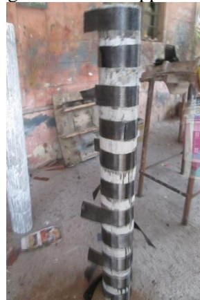
Figure 6. CFRP sheet application (band wrap)
