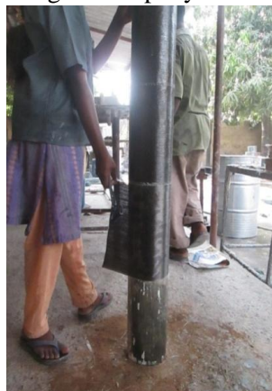
Figure 5. CFRP sheet application (full wrap)
